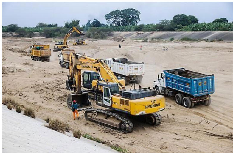
Picture 10. Dredging of the riverbed in the northern part of Peru
